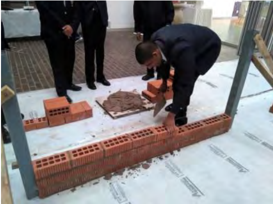
Pranav Gopal laying a brick on a non-loadbearing wall
