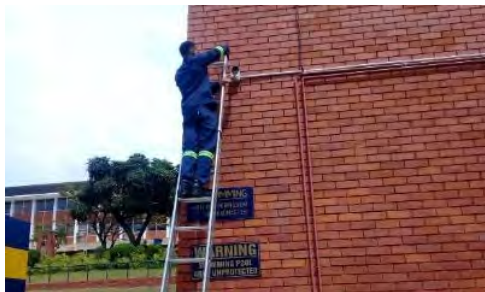
Installing a security camera
