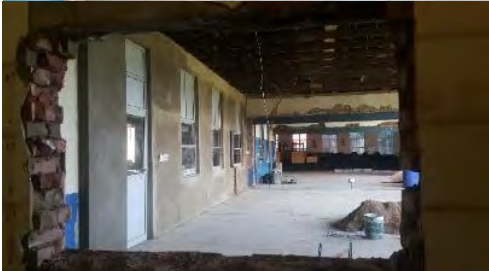
The Nonpareil Cambridge Academy upgrade in progress
