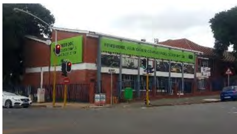
The Newbridge upgrade in progress
