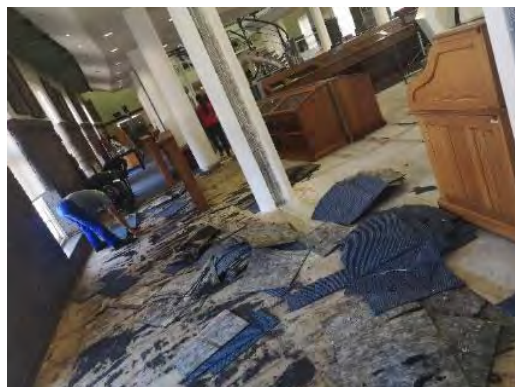
Old carpets being pulled up and the brand new ones going in
