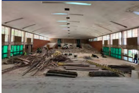
Upgrade of the School Hall in progress
