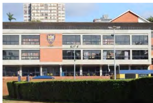
The new solar system was installed on the roof of the new REM Building
